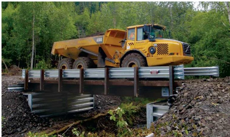
Photo 2-2. Example of Prefabricated, Modular Steel Vehicle Bridge
