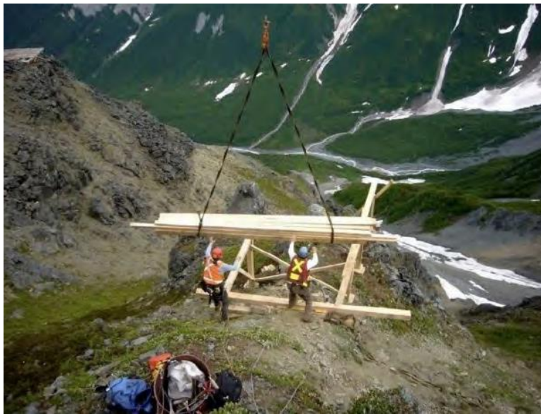
Photo 2-3. Slinging Decking Material for Drill Pad Construction
